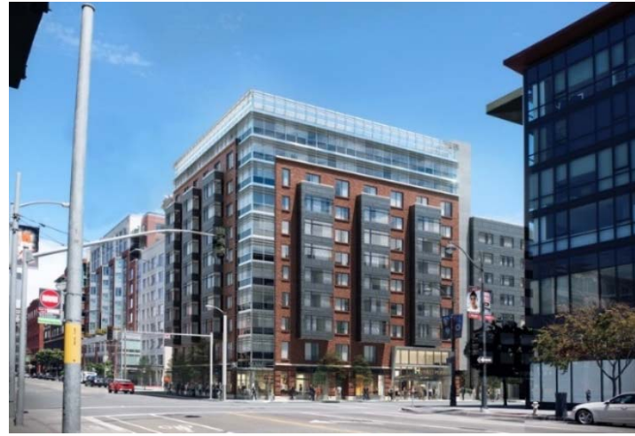
Hyatt Place San Francisco (under construction)
